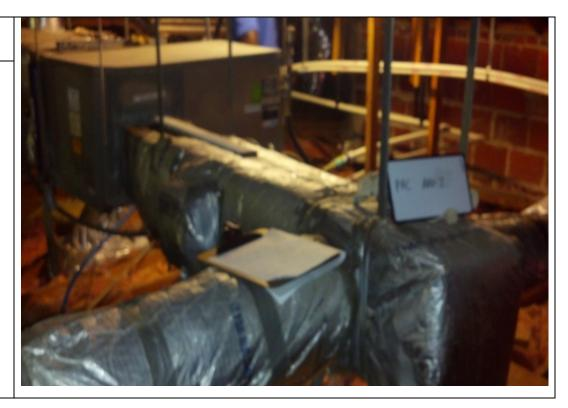
Typical hanging arrangement for AHU 2-4 and 2-5
